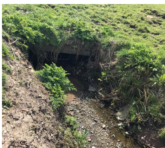
Image 7: Culvert number 4 north to the railway line, which proposed to be replaced
