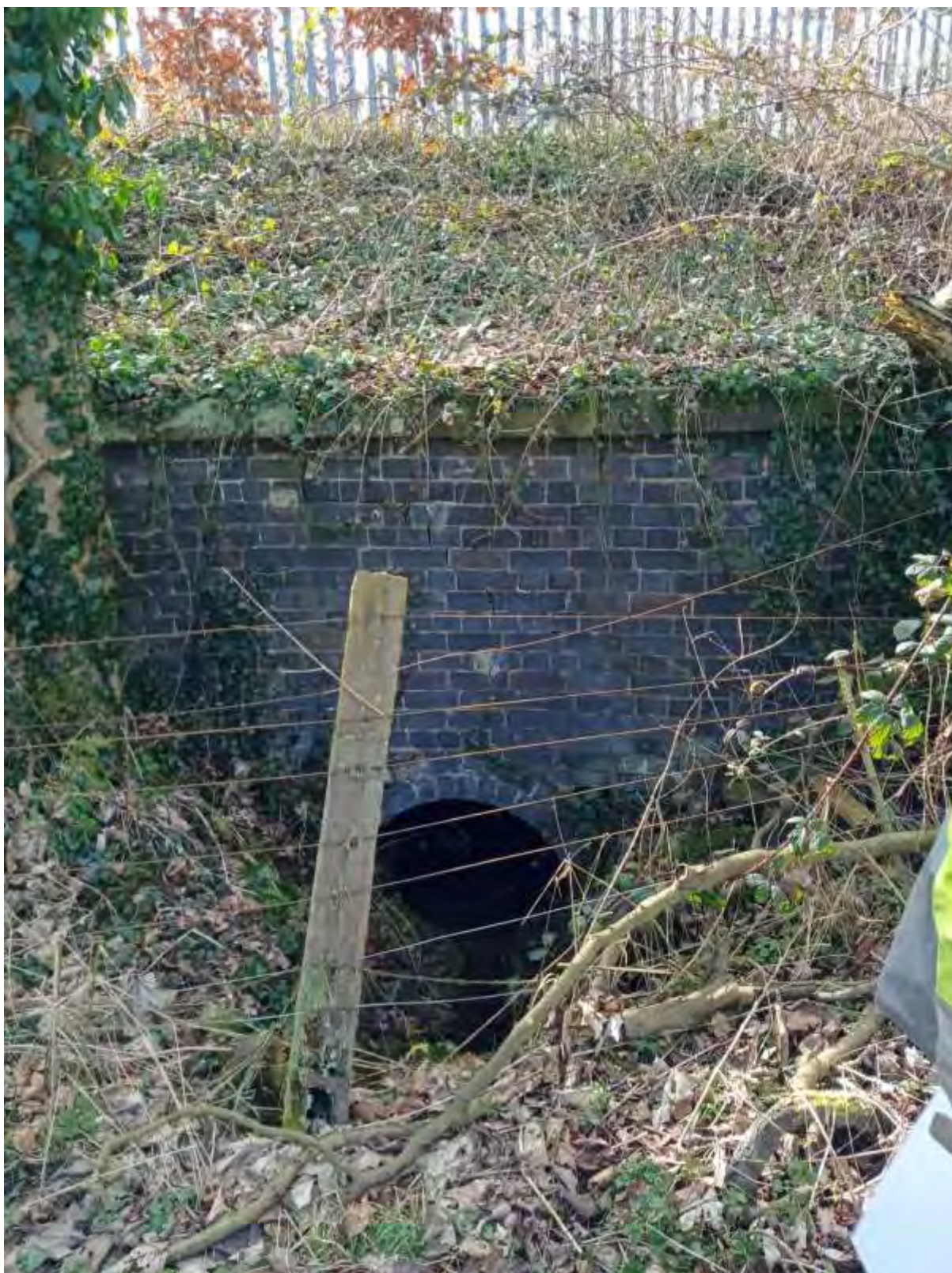
Culvert where stream runs underneath railway. One large crack is noted from the crest of the arch to the top of the bridgework.
