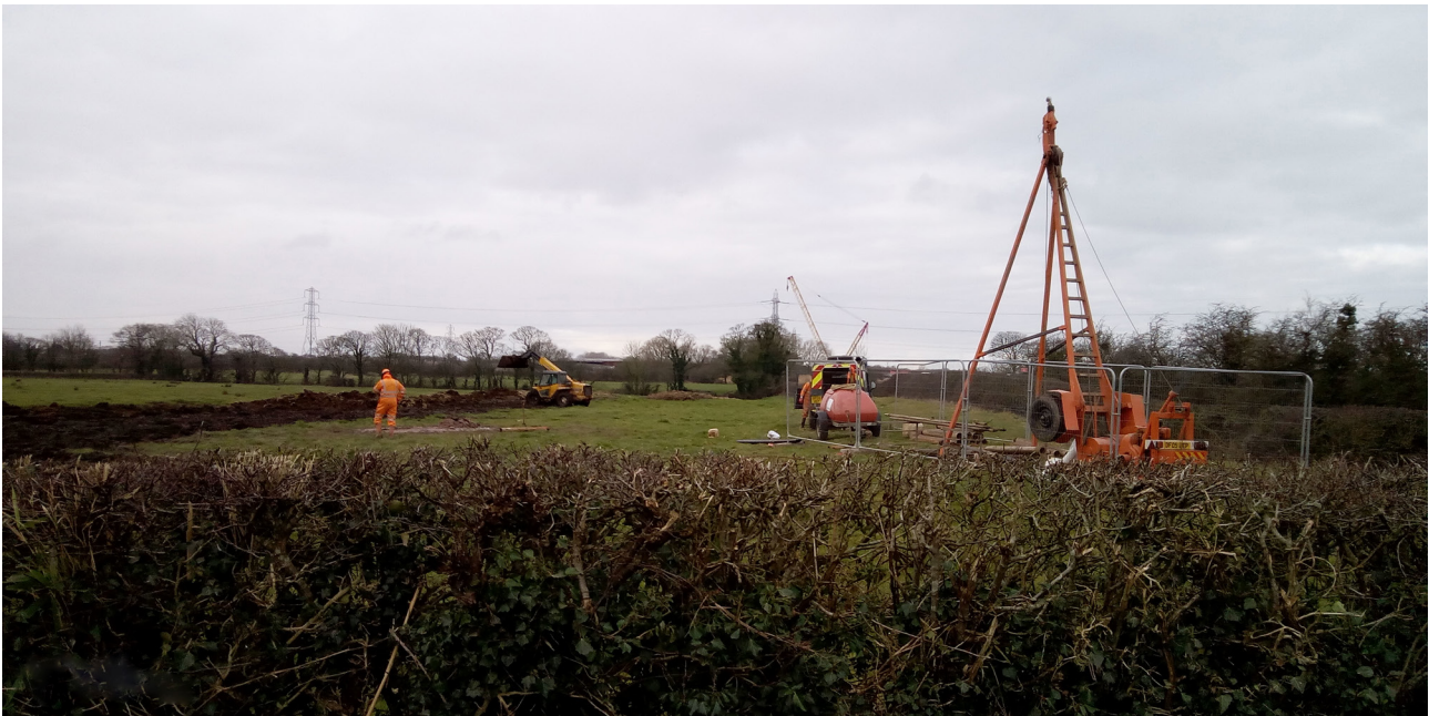
ILLUS 3 F3, looking west
