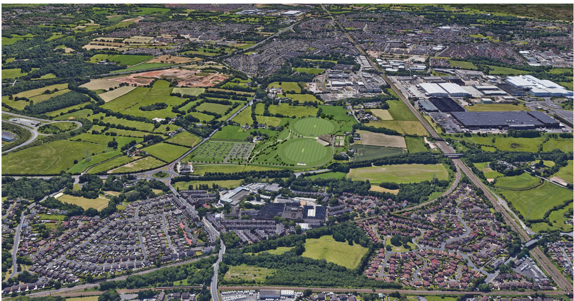
Figure 5.2: Aerial View of the Site from the North - Proposed
