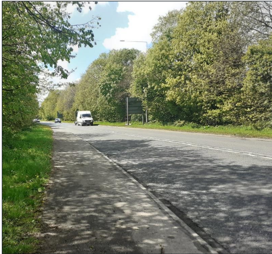
Figure 2-4 - The A582 west of its junction with Stanifield Lane (Facing west)
