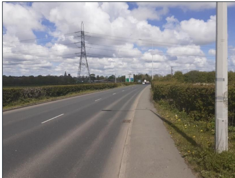
Figure 2-2 - Stanifield Lane by Stoney Lane (Facing North) 1
