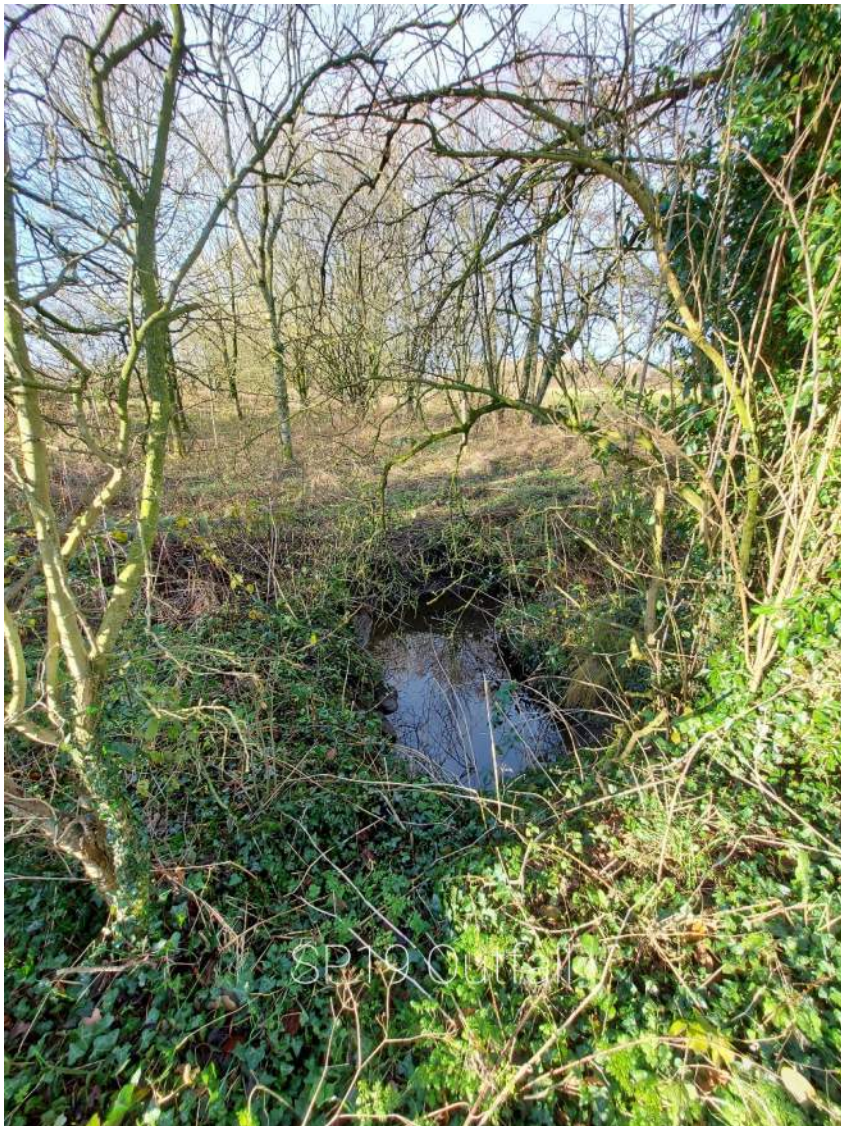
Outfall away from site
