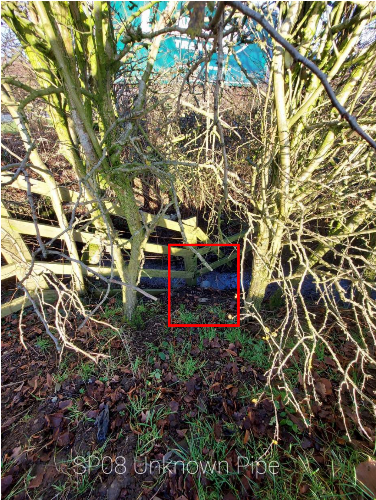
Unknown pipe found out falling into SP 08 ditch. The pipe carried constant flow with the head of the pipe unfound. Assumed to be land drainage. Exposed vertical open pipe found in the field upstream of discovered pipe (See vent pipe 02 image and General arrangement for location).
