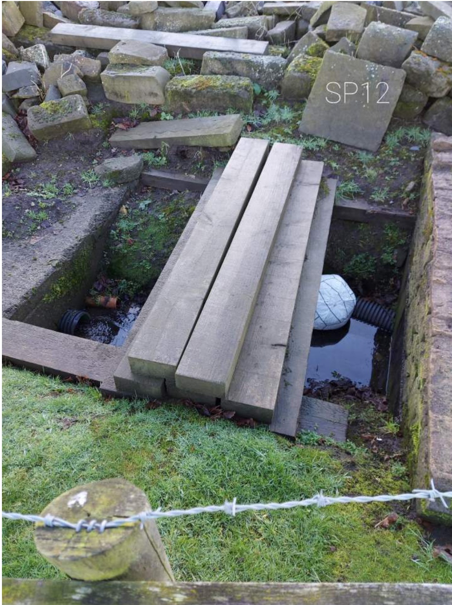
The sheep dip contained ponded water. No flow visible. The team was unable to retrieve a depth from this location.
