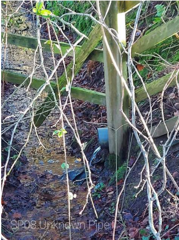
Continuous flow visible of unknown pipe.
