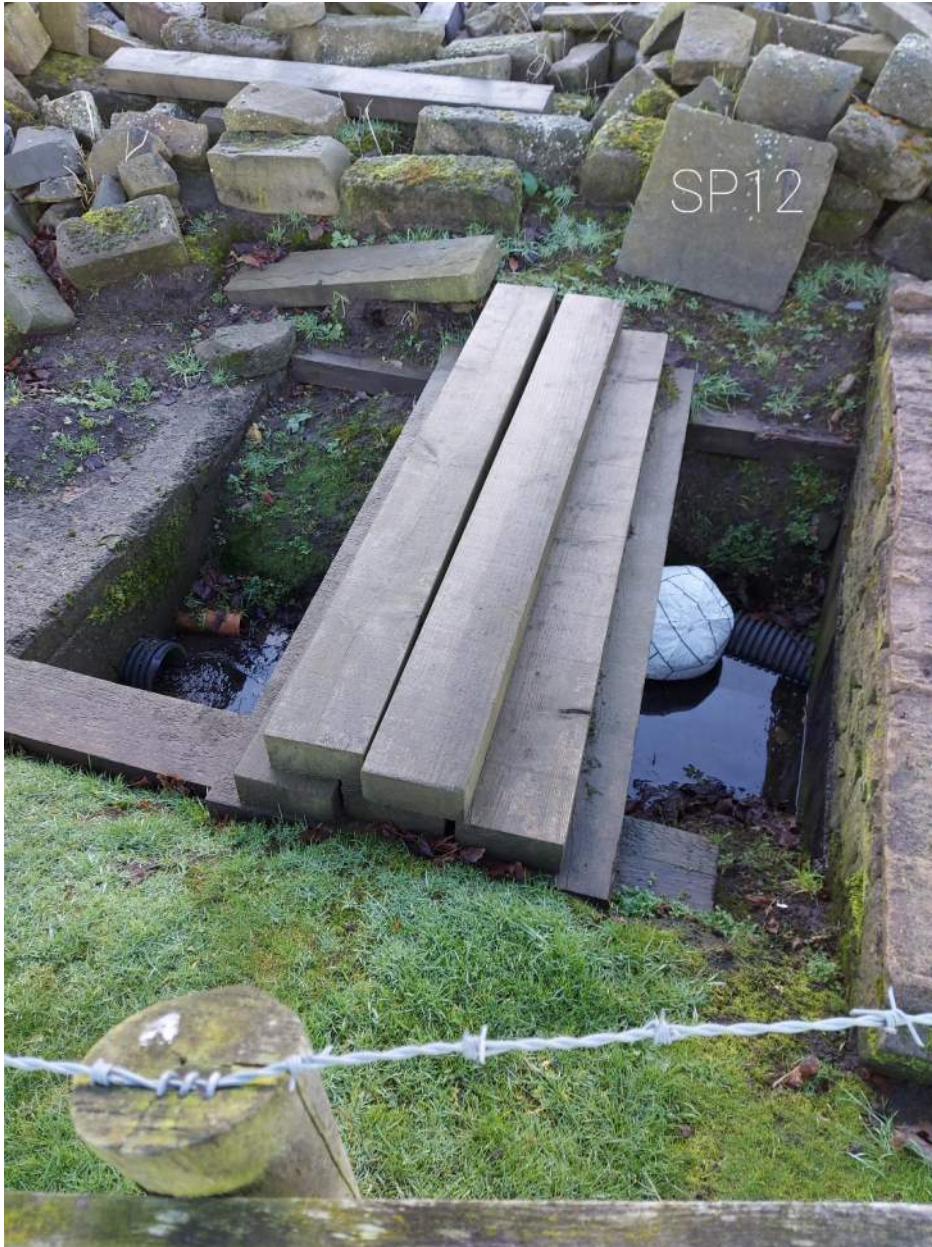
The sheep dip contained ponded water. No flow visible. The team was unable to retrieve a depth from this location.
