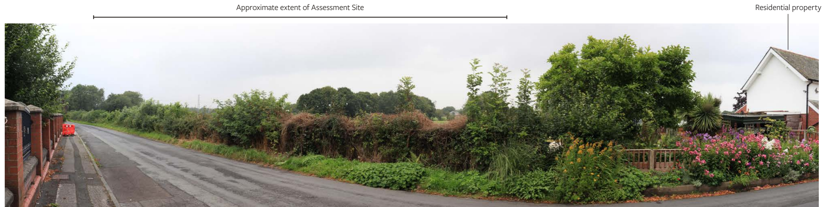
Viewpoint 2 (visible) - View looking north east towards the Site from Fowler Lane, close to Yew Tree Farm, located approximately 125m from the Site boundary. Views towards the Site from this location are almost entirely screened by intervening vegetation along Fowler Lane and along the southern Site boundary. Some limited, close-range, glimpsed and filtered views are available towards and over the southern area of the Site, although views into the Site itself are negligible.
