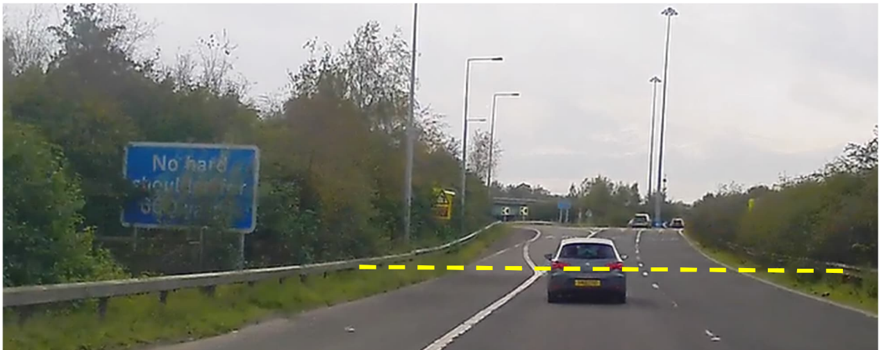
Figure 4-1 - Approximate distance of signals warning signs indicated, where they may be obscured by vegetation or by the “no hard shoulder” sign, and may obscure the bend and roundabout warning signs.
