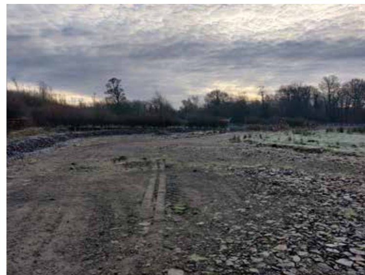
Presumed Temporary Haulage Road leading to Northern Site Access from Wigan Road. Looking East.
