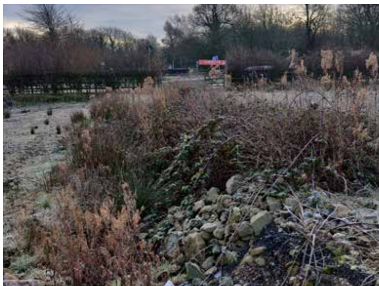
Potential land drain along temporary access road by Northern Site Access from Wigan Road. Looking East.
