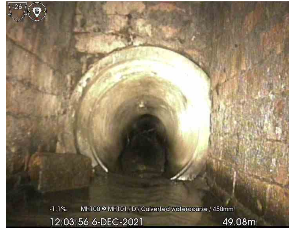
MH100X_49-08m_120356.jpg, 00:05:28, 49.08 m General remark, Buried Chamber
