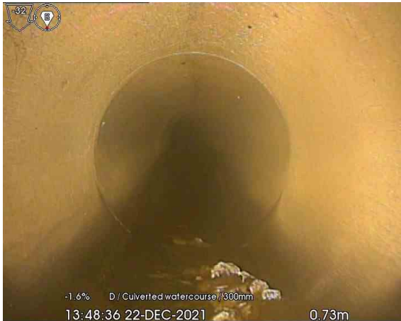
MH6X_0-73m_134836.jpg, 00:00:11, 0.73 m Material changes to concrete
