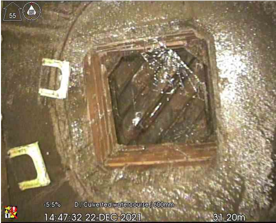
MH7X_31-20m_144732.jpg, 00:02:23, 31.20 m Finish node type, manhole, reference number: MH109
