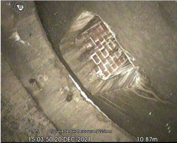
DITCH4X_10-87m_150350.jpg, 00:01:58, 10.87 m Finish node type, manhole, reference number: MH115
