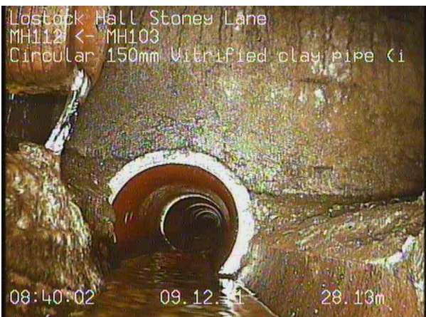
MH112X_6d781c58-cf6e-4bf9-8922-7a11c95af662_20211209_084433_393.jpg, 00:06:19, 28.13 m Finish node type, manhole, reference number: MH112
