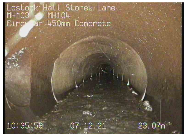
MH103X_f8f7a3ba-4002-4e28-afcf-20d8a8f41735_20211207_093946_650.jpg, 00:02:50, 23.07 m Junction at 9 o'clock, diameter: 150mm, GY1
