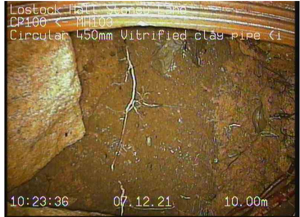
CP100X_92486448-f017-468f-89e5-167630283eec_20211207_092724_566.jpg, 00:03:22, 10.00 m Soil visible beyond defect
