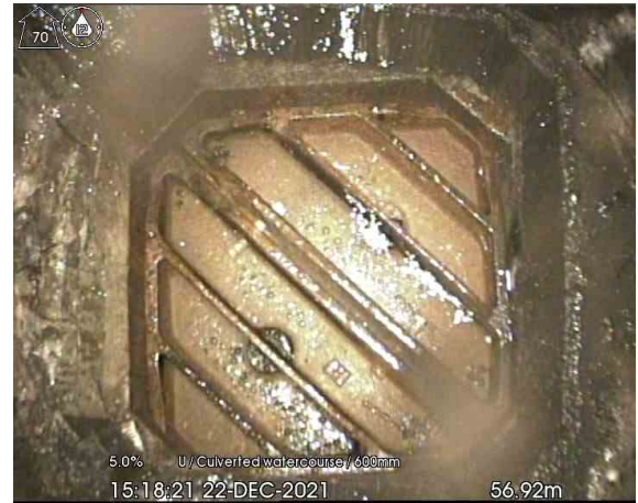
MH09X_56-92m_151821.jpg, 00:03:53, 56.92 m Finish node type, manhole, reference number: MH09
