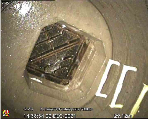
MH108X_29-12m_143834.jpg, 00:02:37, 29.12 m Finish node type, catchpit, reference number: CP4
