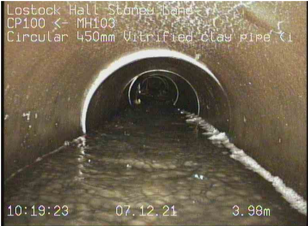
CP100X_2fba9b8d-ee7a-4bca-b569-5b92df62eada_20211207_092310_652.jpg, 00:00:29, 3.98 m Water level, 40% of the vertical dimension
