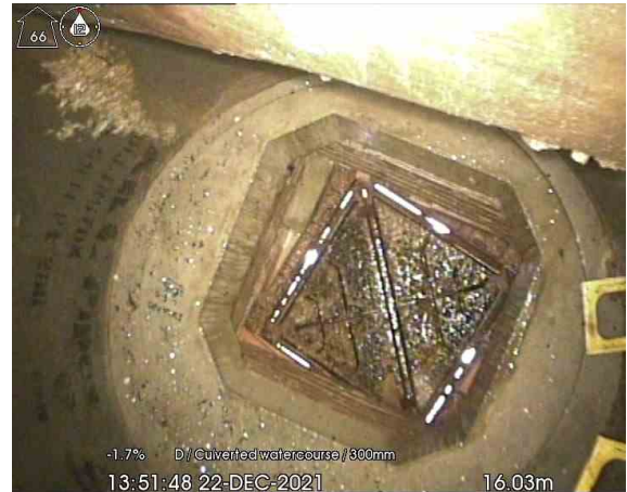
MH6X_16-03m_135148.jpg, 00:02:18, 16.03 m Finish node type, manhole, reference number: MH108
