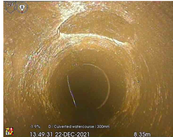
MH6X_8-35m_134931.jpg, 00:00:59, 8.35 m Connection other than junction, closed, at 12 o'clock, diameter: 150 mm
