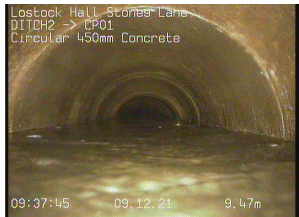
DITCH2X_f3ed88de-811e-4aae-a13e-beadc7fd6f69_20211209_094216_741.jpg, 00:01:41, 9.47 m Water level, 50% of the vertical dimension
