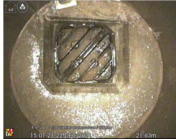
MH109X_21-63m_150121.jpg, 00:01:32, 21.63 m Finish node type, manhole, reference number: MH110
