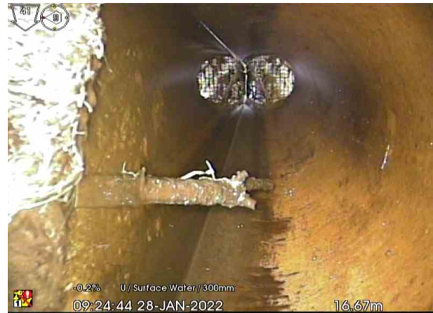
UPSTREAMX_13339ec1-e0c3-4883-af2d-2229c20abef1_202 20131_072141_065.jpg, 00:01:53, 16.67 m General photograph taken at this point, Connection from field
