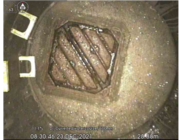
MH110X_28-88m_083046.jpg, 00:02:22, 28.88 m Finish node type, manhole, reference number: MH111
