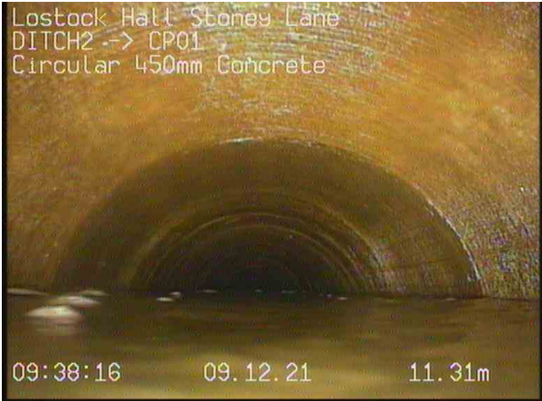
DITCH2X_55b7e539-8cd4-4388-bfe9-305bde17a0a0_20211209_094247_657.jpg, 00:02:06, 11.31 m Water level, 60% of the vertical dimension
