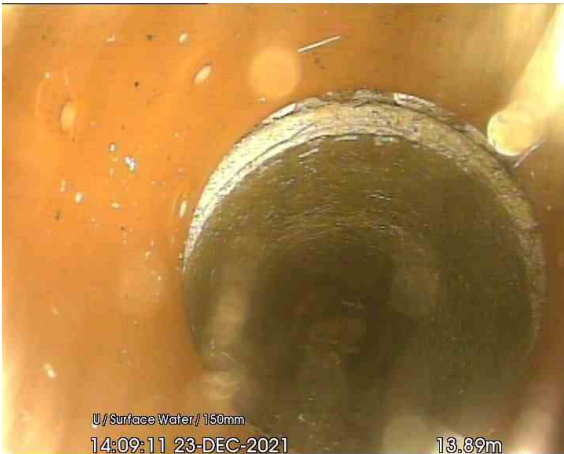
CP3 PIPE D_13-89m_140911.jpg, 00:01:13, 13.89 m Material changes to concrete
