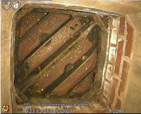
DITCH5X_8-22m_102315.jpg, 00:01:09, 8.22 m Finish node type, manhole, reference number: MH117
