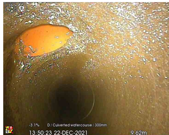
MH6X_9-62m_135023.jpg, 00:01:19, 9.62 m Connection other than junction, at 11 o'clock, diameter: 150 mm
