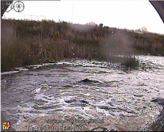
DITCH6X_11-15m_104327.jpg, 00:00:57, 11.15 m Finish node type, outfall, reference number: POND1
