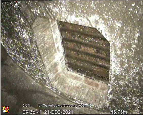
MH116X_45-73m_093641.jpg, 00:03:07, 45.73 m Finish node type, manhole, reference number: MH116
