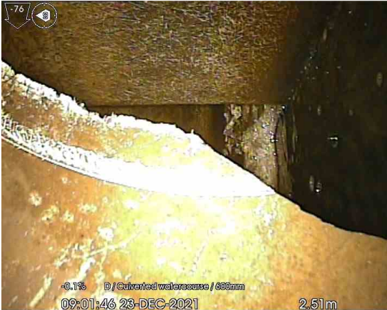
MH112X_2-51m_090146.jpg, 00:01:21, 2.51 m Finish node type, outfall, reference number: OUTFALL, Syphon
