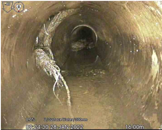
MH102 Upstream_16-00m_092430.jpg, 00:01:37, 16.00 m Connection other than junction, at 10 o'clock, diameter: 150 mm
