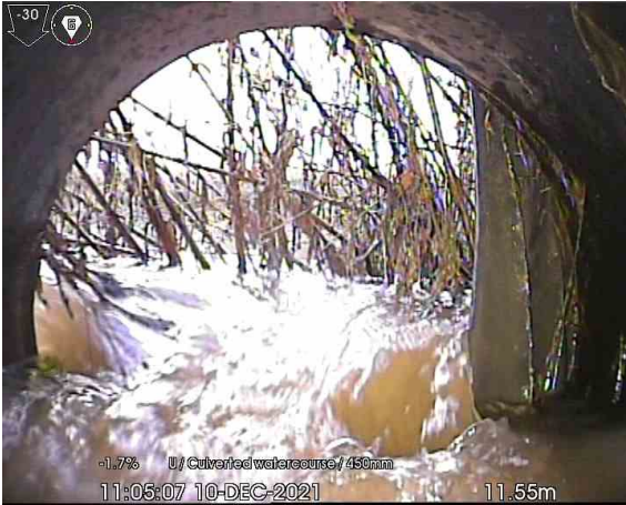
POND1X_11-55m_110507.jpg, 00:01:46, 11.55 m Finish node type, outfall, reference number: POND1
