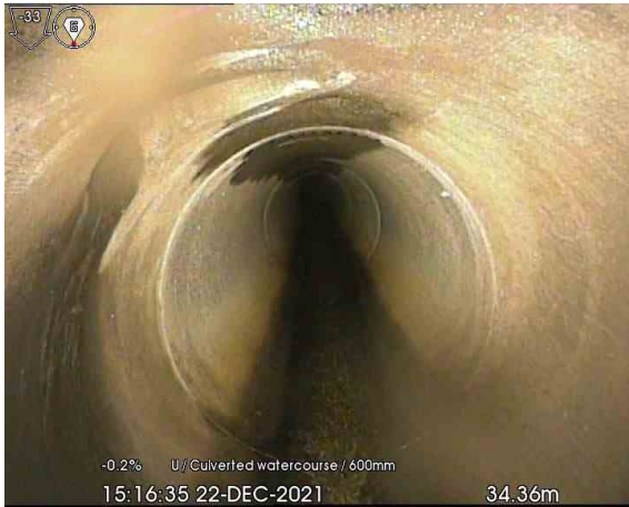
MH09X_34-36m_151635.jpg, 00:02:13, 34.36 m Connection other than junction, at 10 o'clock, diameter: 150 mm
