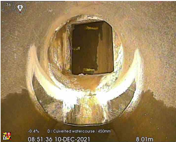
MH114X_8-01m_085136.jpg, 00:00:50, 8.01 m Junction, at 06 o'clock, diameter: 450 mm
