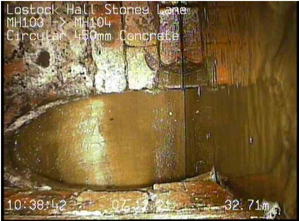
MH103X_21f349de-3db2-48c6-b839-7195f9f8e13c_20211223_150922_926.jpg, 00:05:24, 32.55 m General photograph taken at this point, 2nd Incoming pipe you can see is coming from MH100X
