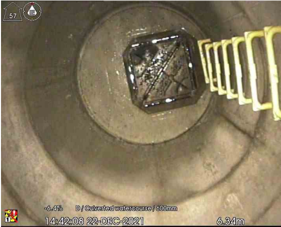
CP4X_6-34m_144208.jpg, 00:00:41, 6.34 m Finish node type, manhole, reference number: MH7
