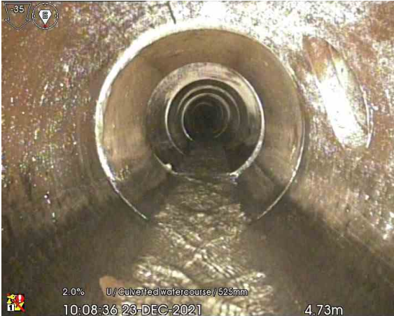
MH104X_4-73m_100836.jpg, 00:00:26, 4.73 m Connection other than junction, closed at 3 o'clock, diameter: 150mm
