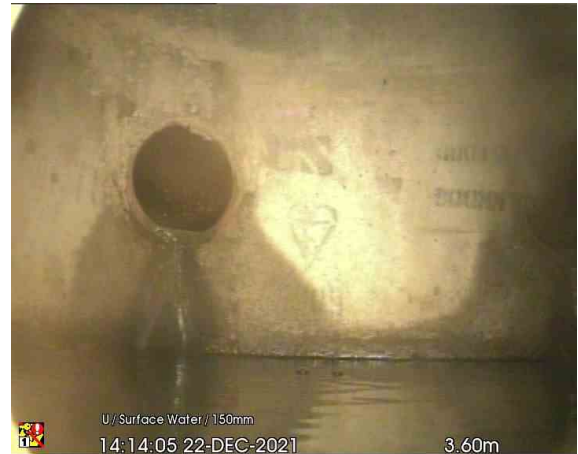
CP3X_3-60m_141405.jpg, 00:00:21, 3.60 m Finish node type, catchpit, reference number: CP3
