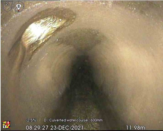
MH110X_11-98m_082927.jpg, 00:01:09, 11.98 m Connection other than junction, at 10 o'clock, diameter: 150 mm
