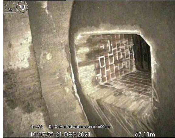
MH117X_67-11m_103755.jpg, 00:06:08, 67.11 m Finish node type, manhole, reference number: MH115
