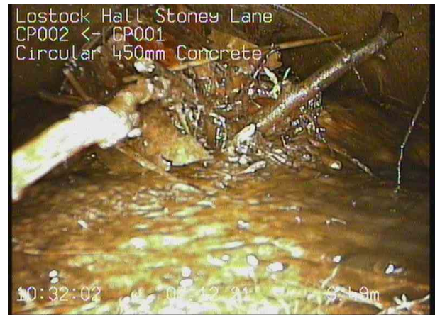
CP002X_7c92932e-6bc4-45c9-a487-1ee05fd42271_20211207_103634_647.jpg, 00:00:45, 3.49 m Survey abandoned, Unable to pass debris
