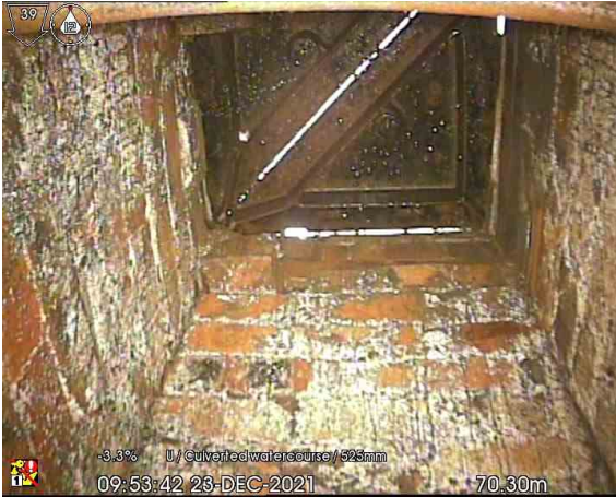
MH105X_70-30m_095342.jpg, 00:07:13, 70.30 m Finish node type, manhole, reference number: MH105
