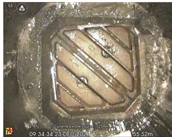
MH106X_55-52m_093434.jpg, 00:07:11, 55.52 m Finish node type, manhole, reference number: MH09
