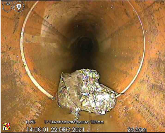
MH3X_26-66m_140801.jpg, 00:04:09, 26.66 m Survey abandoned, Can no longer push rock any further. The rock is getting stuck on the joint.
