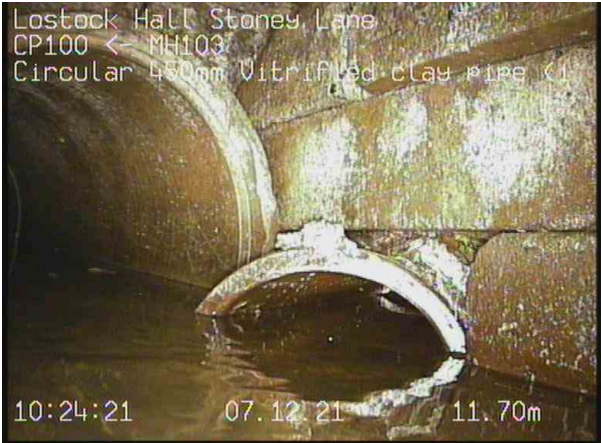
CP100X_06a60654-8b85-4c90-b692-e7a0a90d8e65_20211207_092809_494.jpg, 00:04:01, 11.70 m Finish node type, catchpit, reference number: CP100
