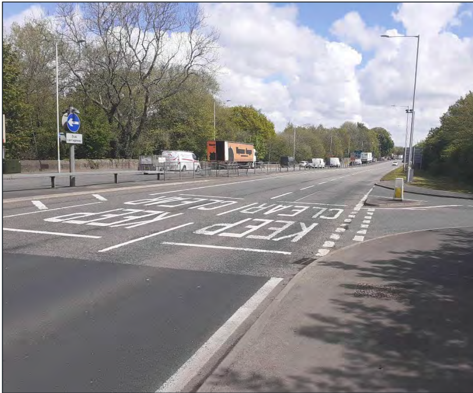
Figure 3-2 - A582 at junction with Old School Lane (Facing East)
