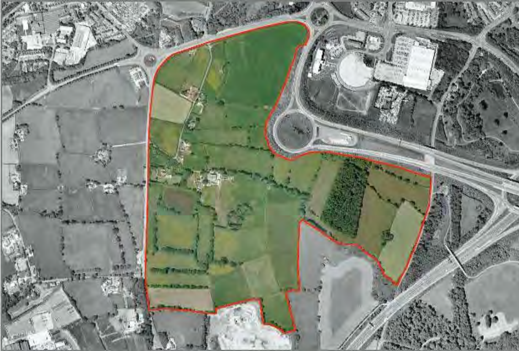
Plate 1: An aerial view of the Cuerden Strategic Site (Image courtesy of Google Earth).
