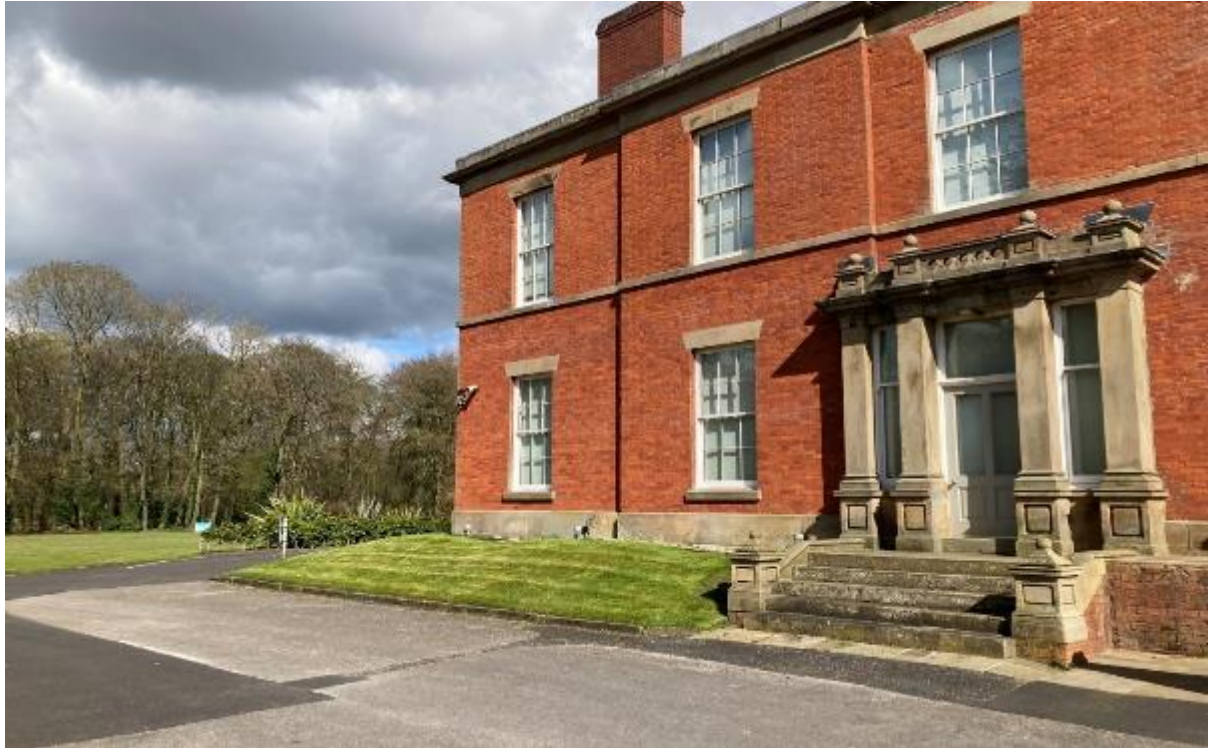
Plate 14: Farington House, facing north-east towards Stanifield Lane
