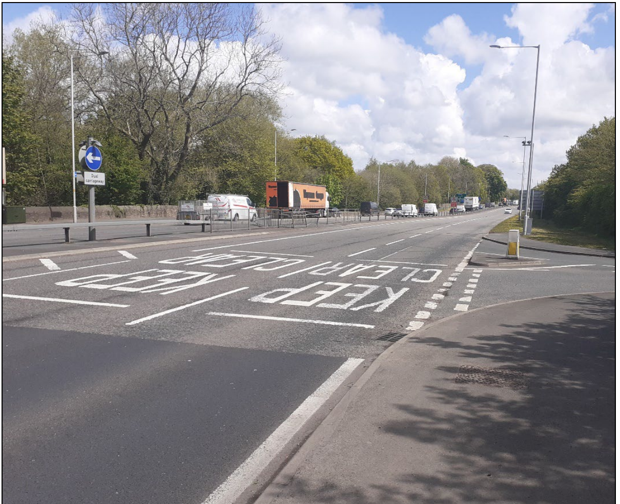
Figure 9.2- A582 at its junction with Old School Lane (Facing East)
