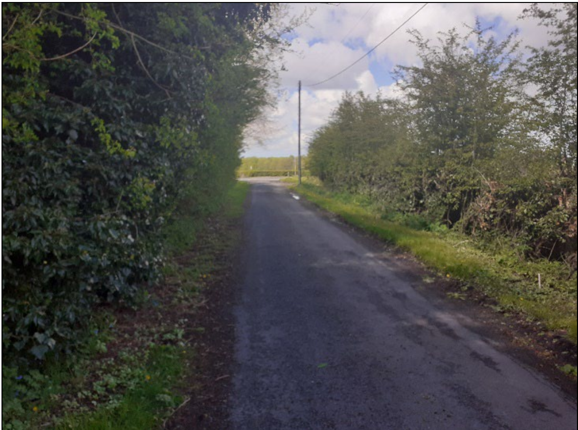
Figure 9.5 - Stoney Lane (Facing West)
