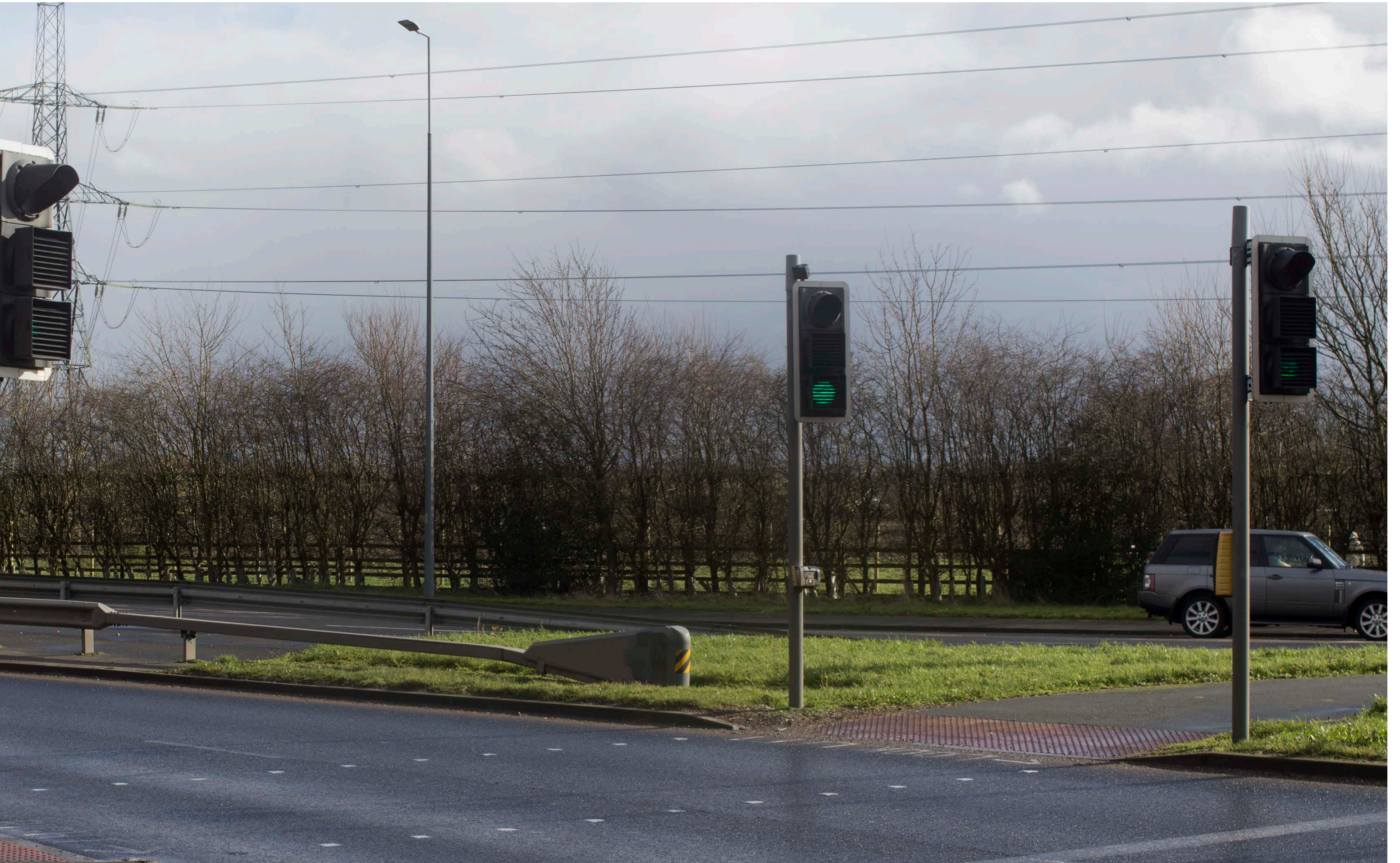
VIEWPOINT 11 SOUTH EAST FROM ROUNDABOUT AT INTERSECTION OF LOSTOCK LANE (A582) AND WATKIN LANE
