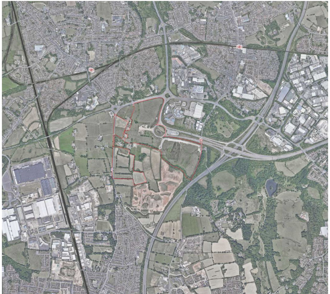
Aerial view of existing site
