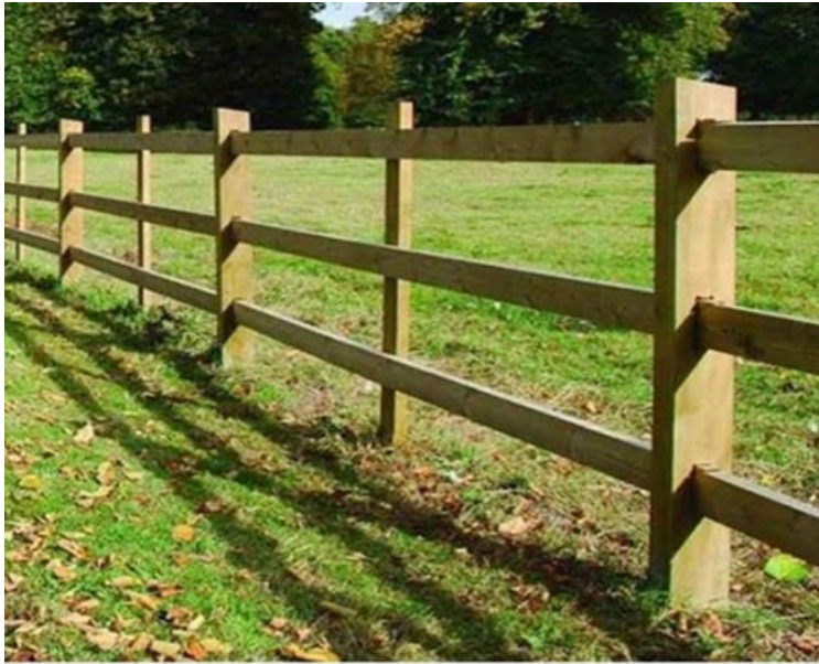
Timber post and rail fence: Caravan park entrance
