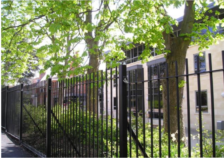
Alpha rail: standard vertical bar steel railings with flat top and square horizontal bars – Penwortham Methodist Church and on top of wall at Ribble Sidings path over embankment
