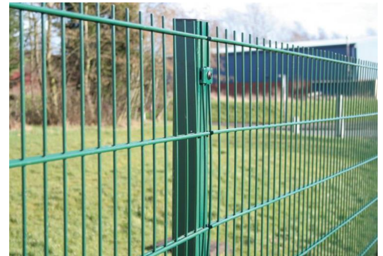
Duex perimeter fencing: 1230mm high around Ribble Sidings wetland habitat
