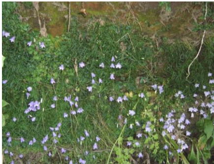
Harebells on part of the river's retaining wall behind the ruin of the 1623 Hall.
