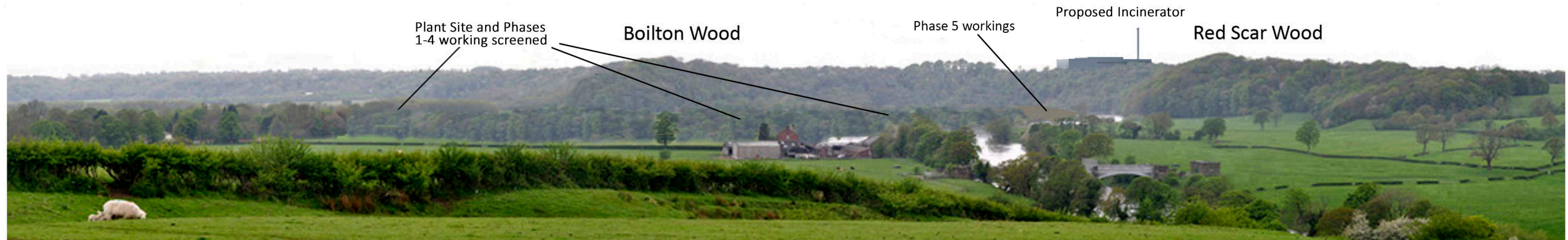
VIEWPOINT 23- as above but with established trees on screen bund at end of Phase 5 Working
