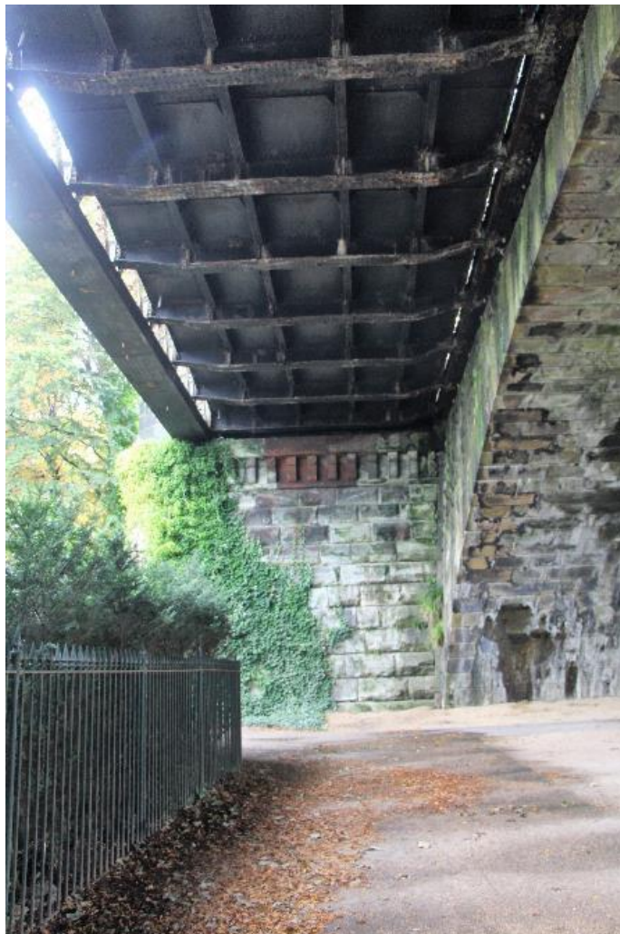
Plate 10 The later 19 th C. widened section of the Railway Viaduct over River Ribble; view from below
