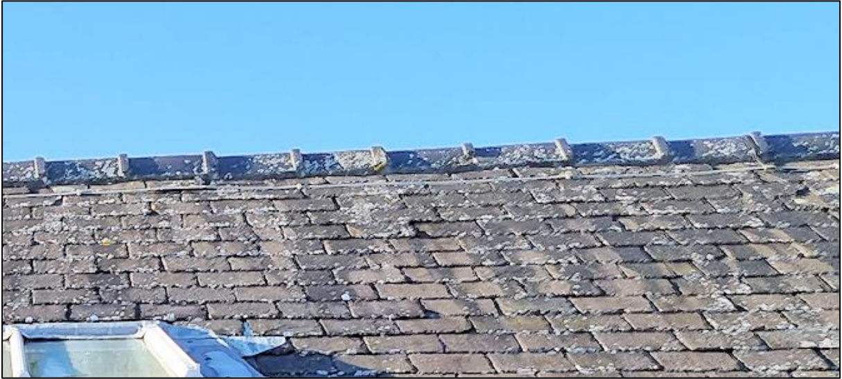
Plate 1: The ridges and roof pitches were intact with no PRFs.
