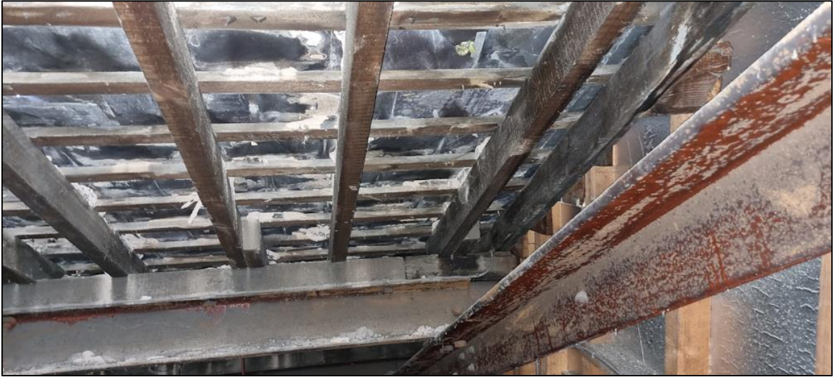
Plate 10: In the voids at the end of each roof, the voids were open to the tiles, the timbers and steel joists.
