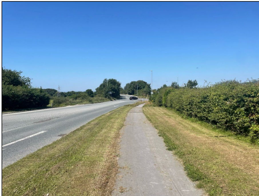
Photograph 9.2: Footways on Kellet Road
