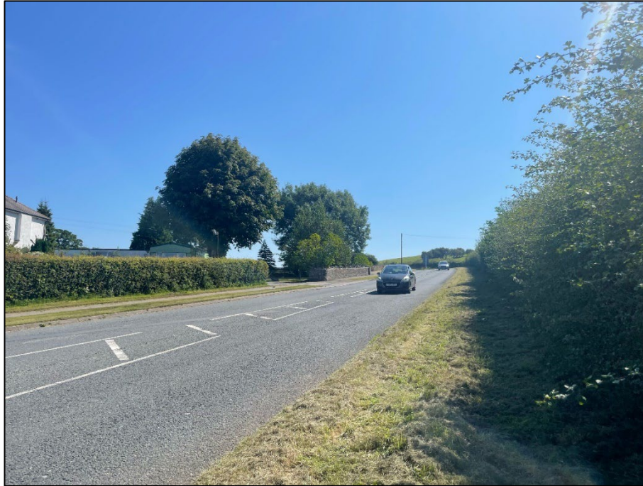
Photograph 9.5: Kellet Road (view to the east of the site)
