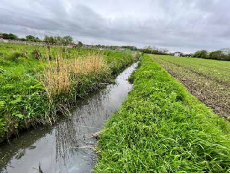
D1- A wide ditch with slow flow to the edge of arable fields
