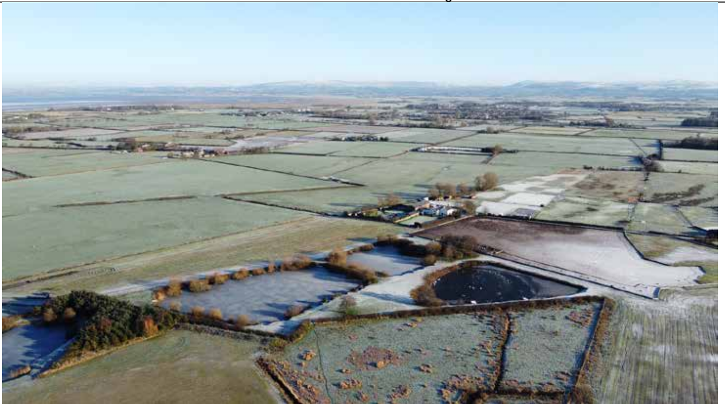
Site from 120m altitude looking North (during cold weather)
