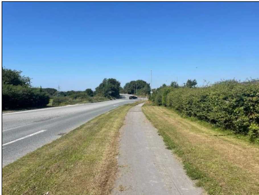
Photograph 2: Footways on Kellet Road
