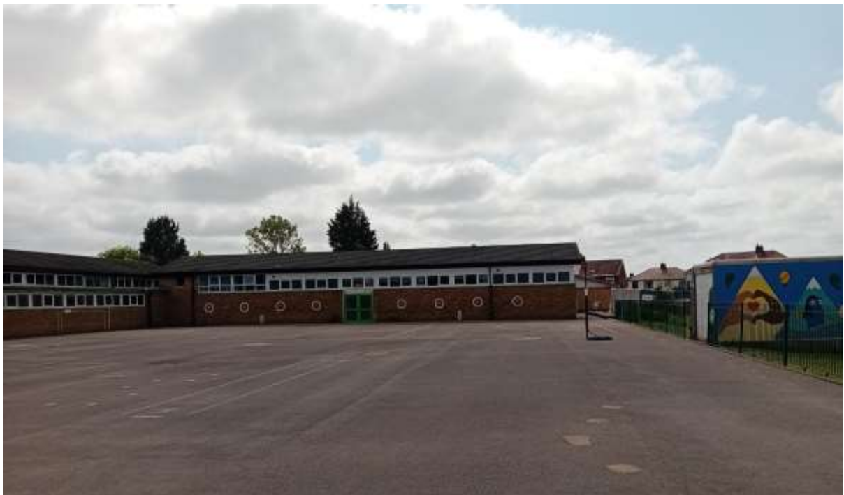
Photo 2:- Existing school playground in a Westerly direction. The proposed new extension to sit on the grass to the right of the playground
