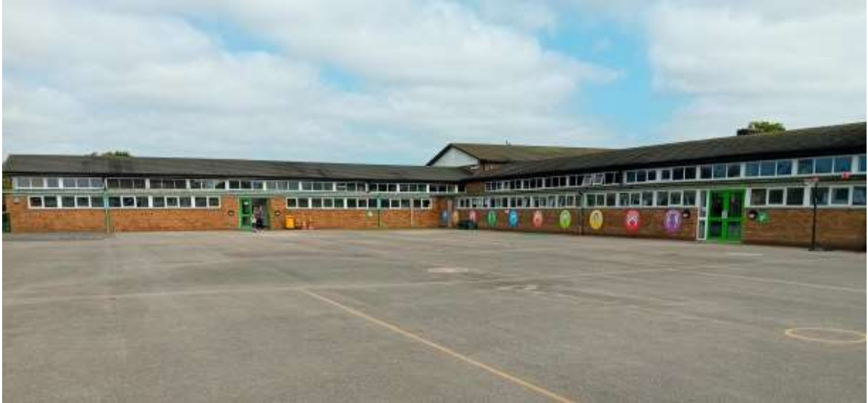
Photo 3:- Existing school playground in an Easterly direction, tarmac playground to be retained in it's entirety.
