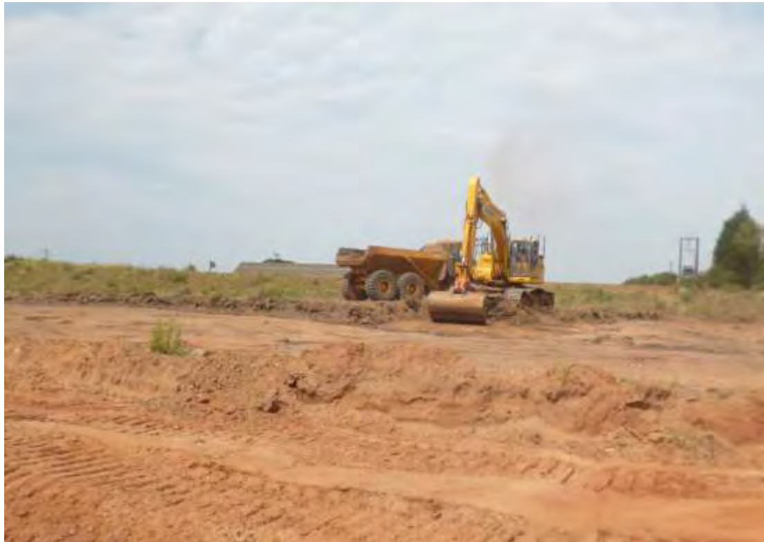
Soil Stripping Process
