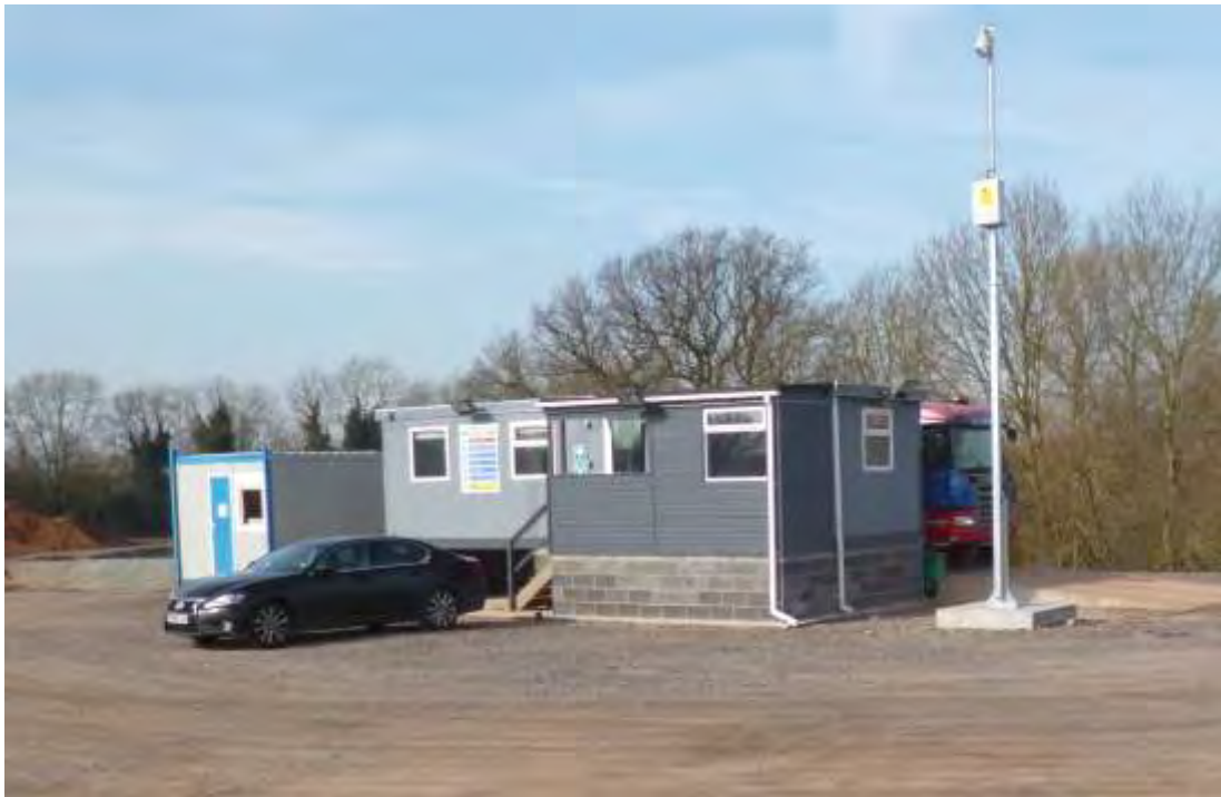
Typical Weighbridge Office
