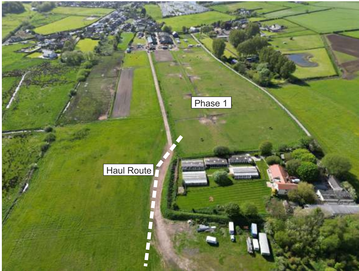
Phase 1 -Looking West
