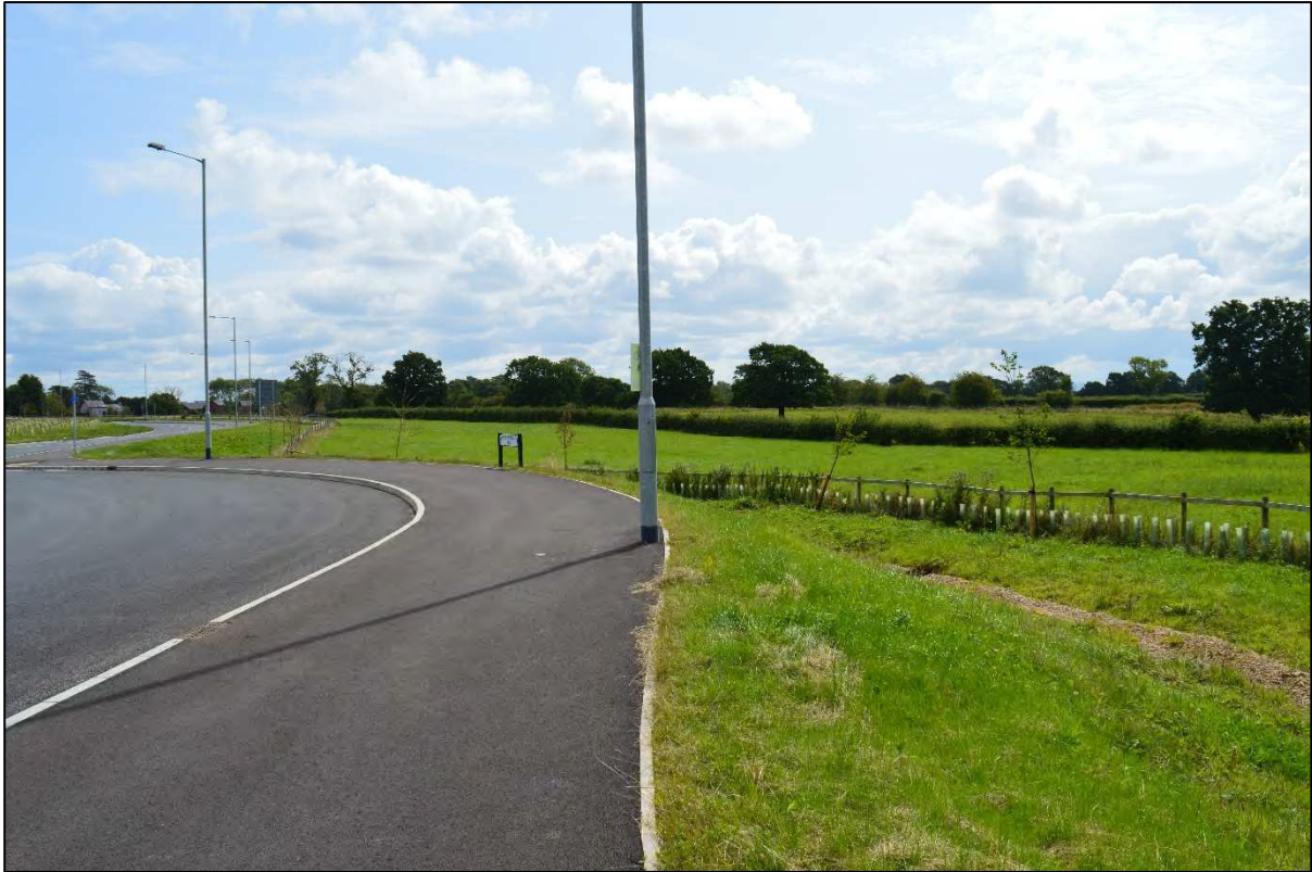
Plate 15: Land south of new roundabout, facing east
