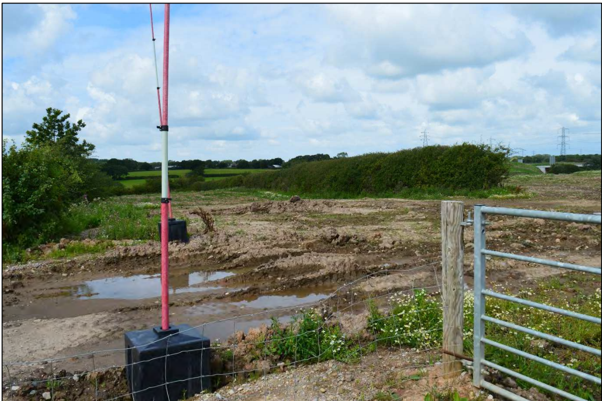
Plate 34: Disturbed area east of cycle path, south of Savick Brook/ the Ribble Link Navigation Canal, facing north
